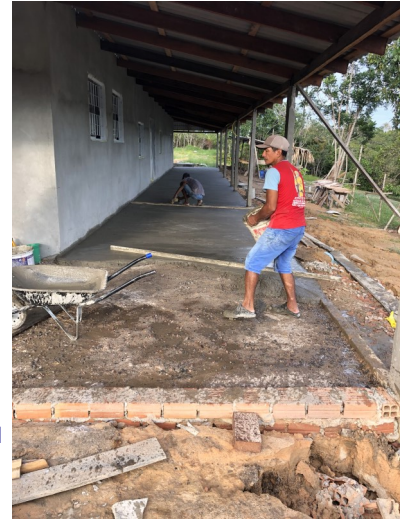
Pouring the front porch!!! The front porch roofing is completed!!!
