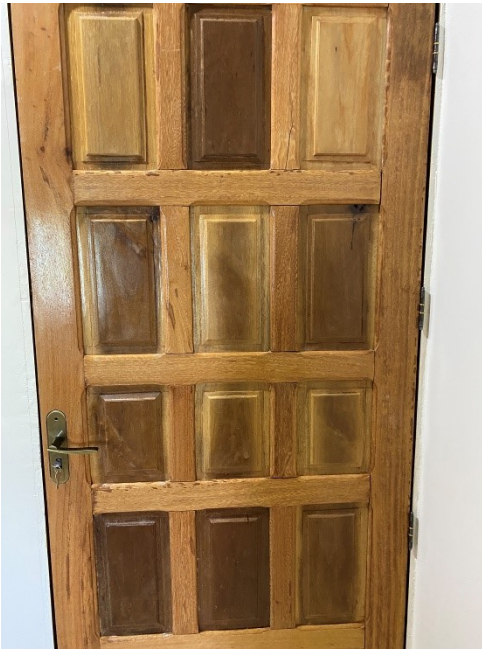
Interior doors installed
