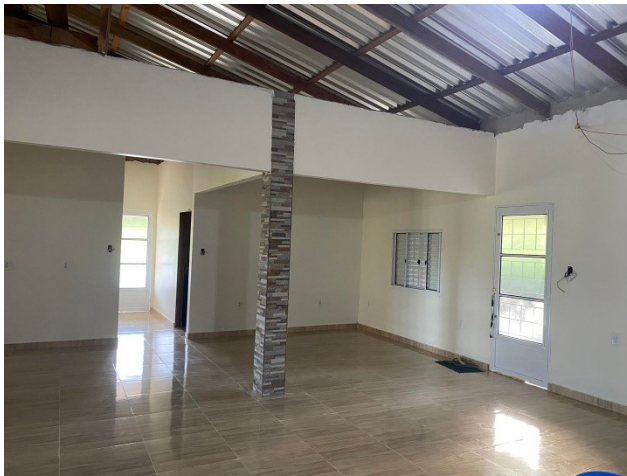
Drop ceiling is being installed
