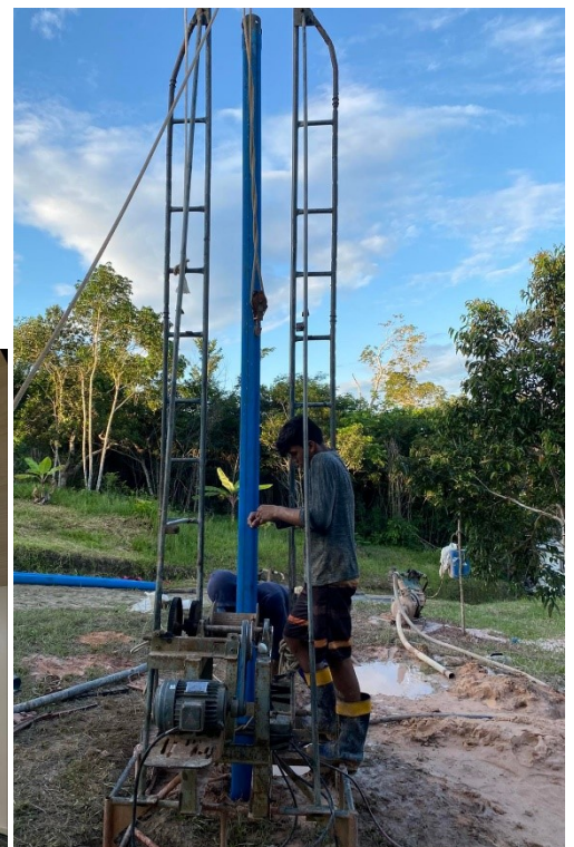
Water well being dug
